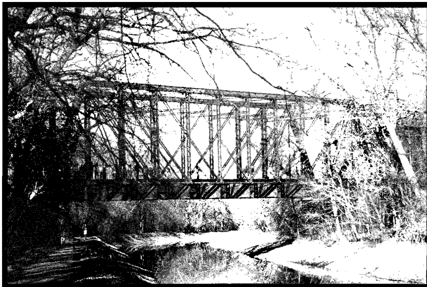
A mighty steel trestle carries the trail over both the C & O Canal and Canal Road at Arizona Avenue. It will be fenced and decked to make it safe for trail use.
