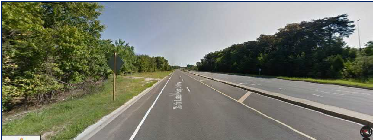
Figure 4 - MD 704 westbound past US 50 Overpass (looking east)
