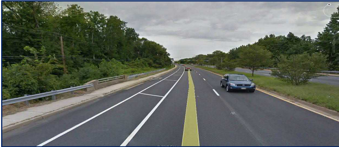
Photo I – Eastbound MD 704, Structure Carrying Cattail Branch (Map Data: Street View, Google)
