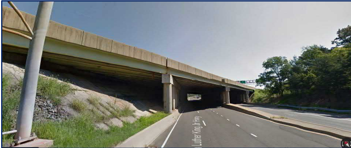
Photo M – Eastbound MD 704, US 50 Overpass (Map Data: Street View, Google)
