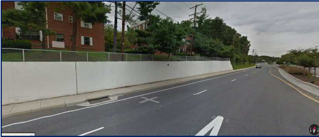
Photo D – Eastbound MD 704, Retaining Wall along Glen Willow (Map Data: Street View, Google)
