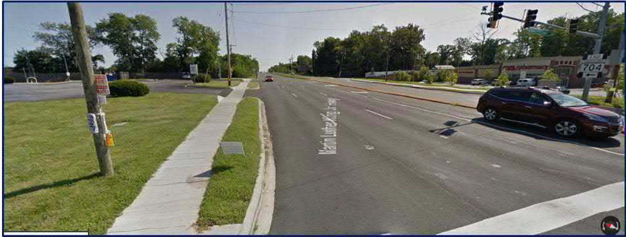
Figure 3 – MD 704 westbound past Ardwick-Ardmore Road (looking east)
