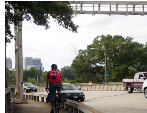
Bicyclists have fallen off this narrow sidewalk on the Roosevelt Bridge into travel lanes (south side looking west)
