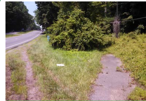
Yet each path or service road ends without connecting anywhere (west of Prosperity Drive, north side)
