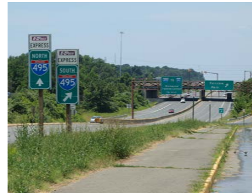
No biking here. Arlington Blvd becomes a limited access freeway as it crosses under I-495.
